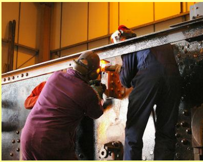
06/08/2010 - Heating rivet and angle support to insert rivet ( Matthew Wilkins' Father )
