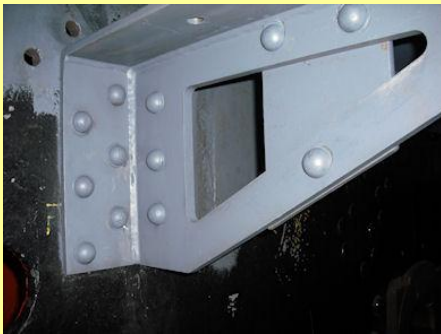
06/08/2010 - Frame angle fully riveted.
