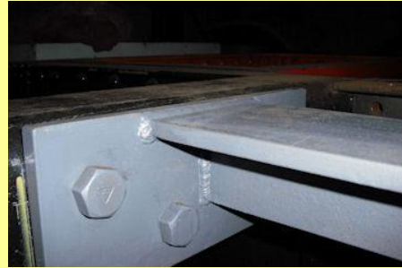
29/05/2010 - Frame angle 19 (the tee bar) repositioned on its end flange and refastened to frame angle 21.
