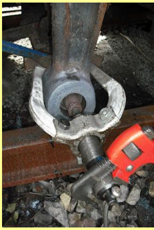
1-2/07/2010 - Puller on H44 bottom boss
