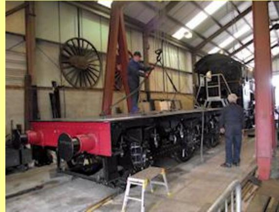
06/09/2017 - fitting the tender base-plate onto the tender chassis.
